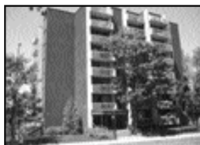
Place du Parc, Quebec City, Quebec
